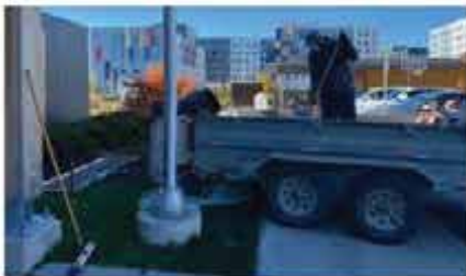
The crew mixing the cement for the cenotaph's foundation.
